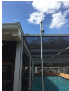
Installed mast and tilt-over base.
